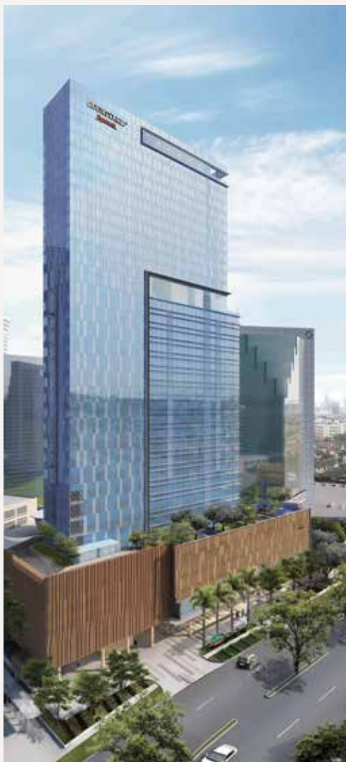
ROYAL SQUARE @ NOVENA Current Project
